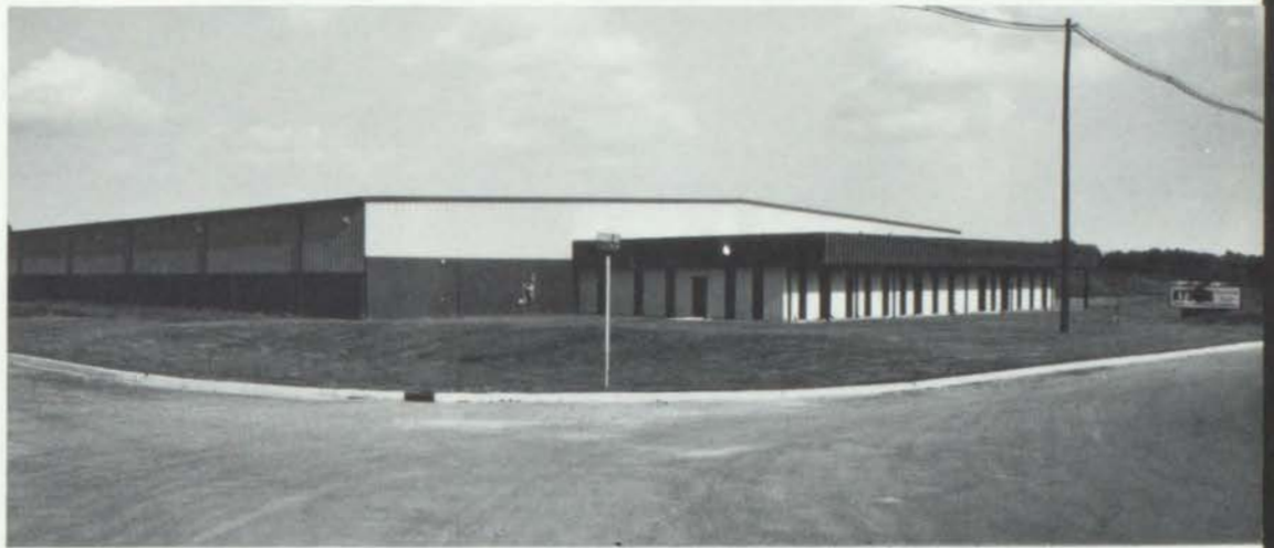
Kysor Machine Tool Division's New Marshall, Michigan plant which was completed and dedicated in August of 1981.
