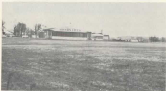
Marshall's airport, Brooks Field.
